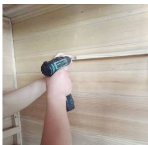
FIG-25 Assemble the towel rack using 2 pcs of 4x25mm screws.
