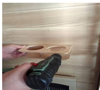
FIG-26 Assemble the cup holders using 2 pcs of 4x25mm screws.
