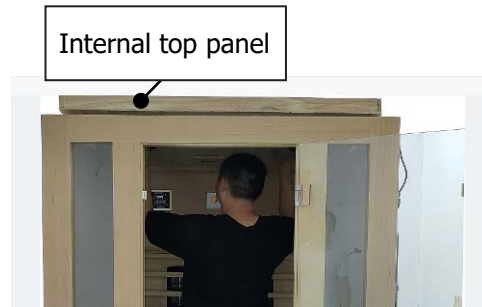
FIG-13 Setting the internal top panel
