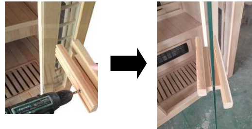
FIG-21 Tighten the screw until it is tight.
