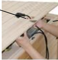
FIG-29 Insert the power plug through the external top panel and use 8 pcs of 4x25mm screws to secure it.
